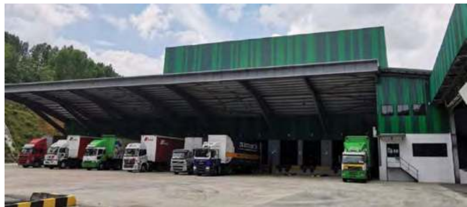
A building with small environmental footprint while providing occupants a healthy & comfortable indoor and outdoor environment. The roof overhang in front of building acts as effective shading device to internal area blocking direct sunlight, further reduce the heat gain in the internal building.
